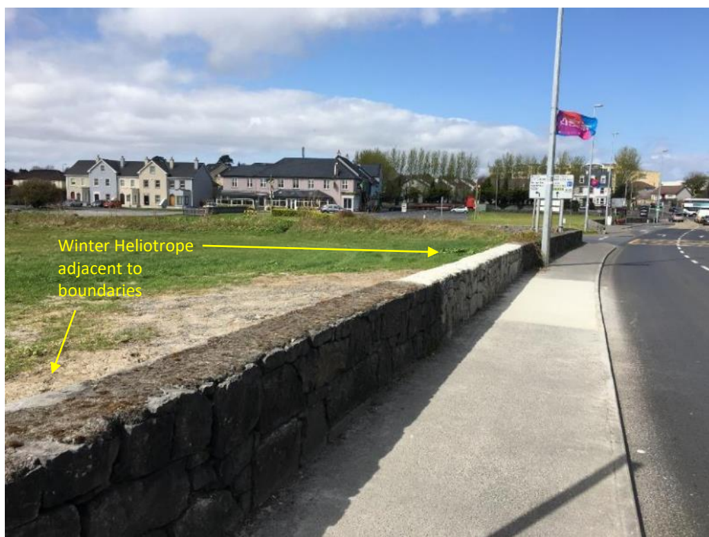
Photo 6. Showing the approach to Moneenageisha junction on the Dublin Road. Note the disturbed ground and wall repairs.
